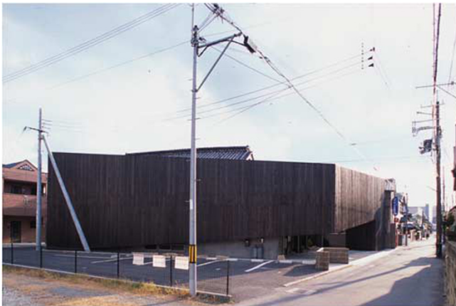
Figure 6 | Exterior of the new element. © Katsuhiro Miyamoto. This image is reproduced with permission of the copyright holder, and is not covered by a Creative Commons Attribution 4.0 International License.
