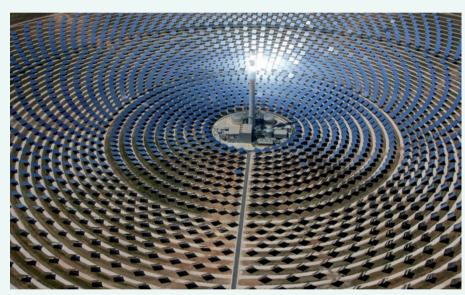
Gemasolar's 19.9 MW turbine is expected to meet the electricity needs of 25,000 Spanish households through the substation of Villanueva del Rey. Were the same amount of energy to be produced by burning fossil fuels, 218,000 barrels of crude oil or 38,600 tons of lignite (low-grade coal) per year would be needed, emitting 30,000 tons of carbon dioxide.
