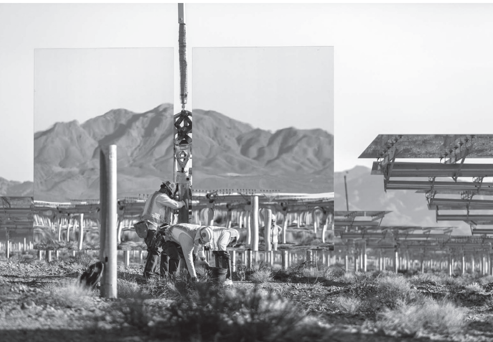
Construction of solar panels in the Mojave Desert, California.
