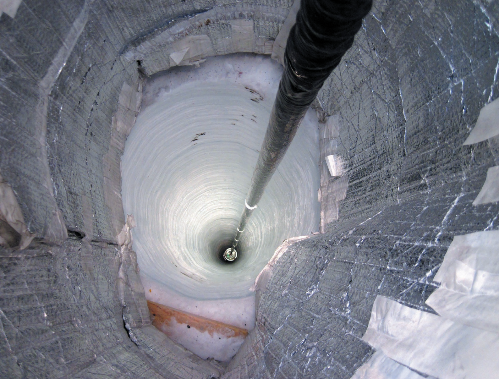
An optical sensor begins its 2,500-metre journey down a borehole to become part of the IceCube neutrino detector in Antarctica.
