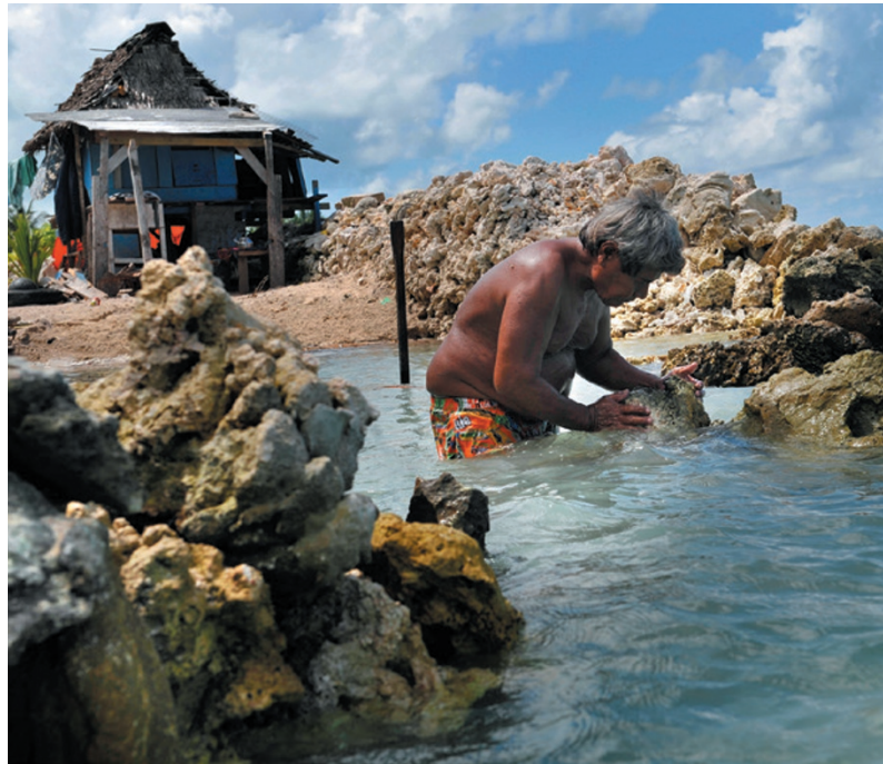
A man rebuilds the sea wall that protects his home on South Tarawa.
