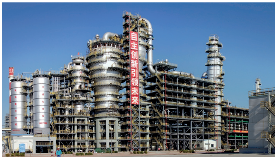
A dimethyl ether/methanol to olefins complex in the Shenhua Baotou plant in Inner Mongolia.
