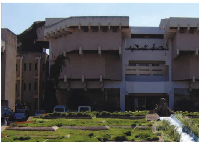
SDM Dental College, Dharwad, India, showing ventilated concrete construction for cooling in the heat of summer.
