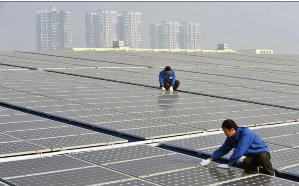
A solar-power plant in Wuhan is part of China's plans to produce 10 billion watts of solar energy by 2020.
