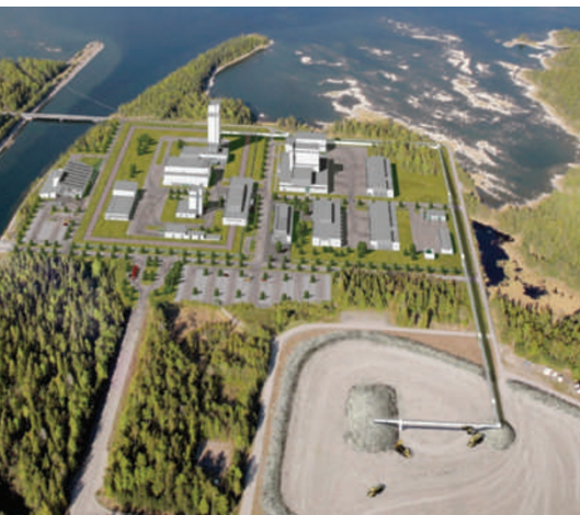
SKE A mock-up of Sweden's nuclear-waste store.
