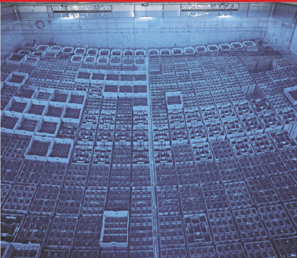
Keep out: storing radioactive waste in surface facilities such as spent-fuel ponds is expensive and risky.
