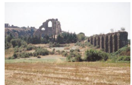
Water works — one of the towers at Aspendos, with (right) remains of the aqueduct.
