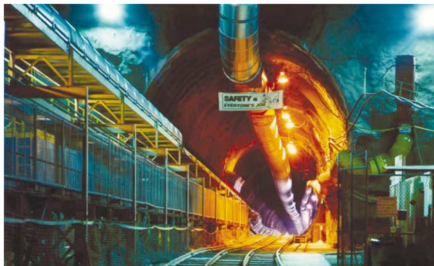
The hole picture: an 8-kilometre tunnel has been bored through Yucca Mountain to allow for tests.
