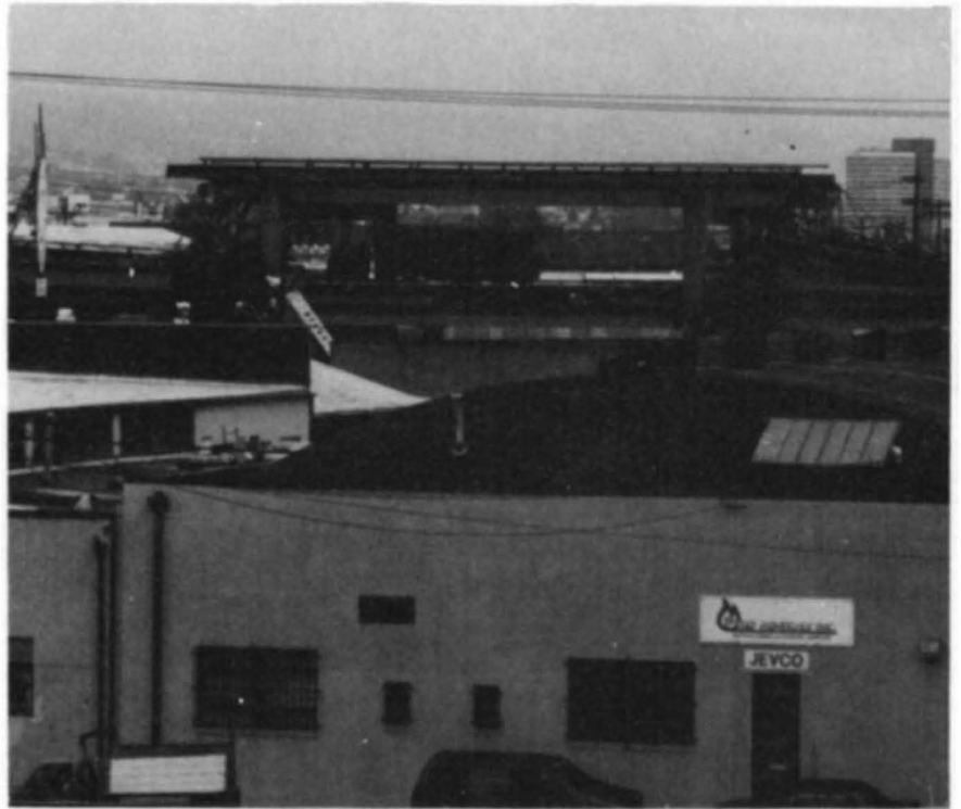
A truck escapes untouched on the lower roadway of the Nimitz freeway in Oakland, California, following the Loma Prieta earthquake of 17 October 1989. In the 1.4-km-long section of the freeway that collapsed in the earthquake, only the segment shown survived; the lower roadway here is supported by three pillars at each end instead of the usual two. On page 853, an analysis of aftershock recordings sheds some light on the failure of the Nimitz freeway; it seems that the presence of three-pillar supports strengthened the segment sufficiently to prevent its collapse.
