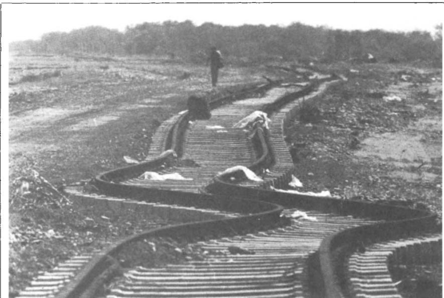
Steel sidewinder — the twisted railroad tracks at Lázaro Cárdenas on Mexico's Pacific coast are a vivid scar left by the earthquake of September 1985, which killed over 9,000 people. The picture is taken from The National Geographic Society — 100 Years of Adventure and Discovery by C.D.B. Bryan, a beautifully presented collection of photographs from the magazine's archives with accompanying commentary. The book is published in the United States by Abrams and in Britain by Phaidon.
