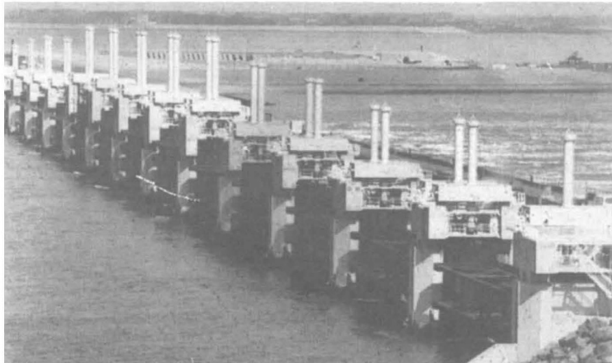
Some of the 63 gates in the Eastern Scheldt barrier. A public road runs along the top of the barrier, 12 metres above sea level.
