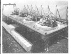
STILL just a model, this is the 16-metre optical telescope, the "Very Large Telescope", planned for the European Southern Observatory (ESO) in Chile. ESO technical committees are now meeting to establish exact specifications for the new instrument with the aim of presenting plans for a DM 300 million project to ESO member countries in time for work to start in 1987. The VLT is to be sited at an altitude of 2,400m, and the human figures in the above photograph put its size into perspective. □
