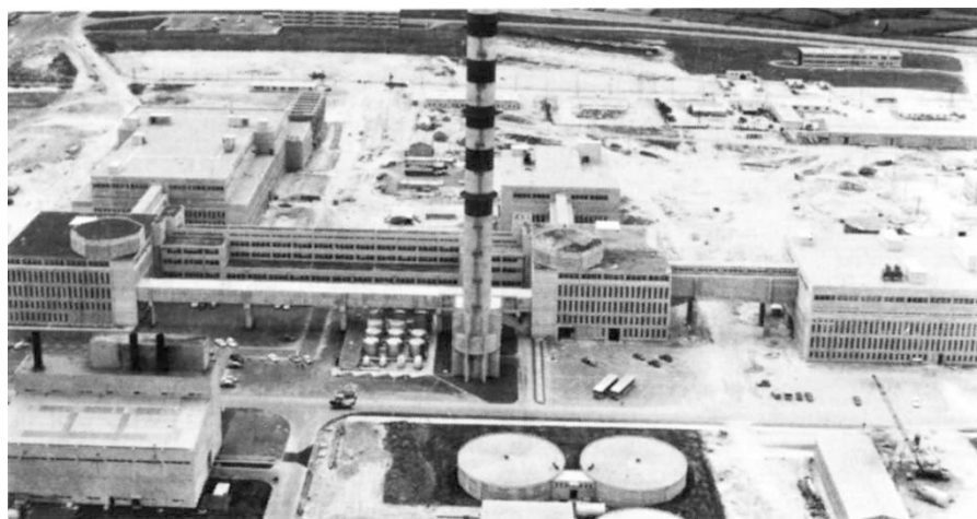
Reprocessing plant at La Hague
