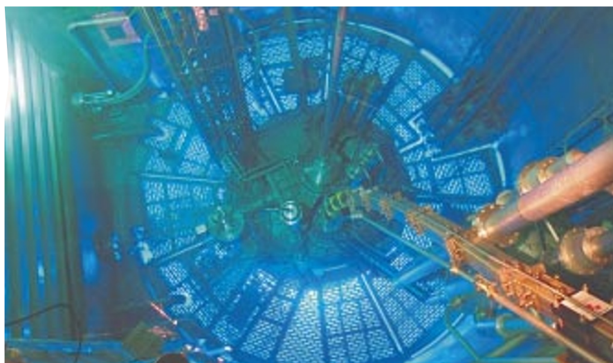
Deep blue: light is emitted from the core of the ILL reactor as a result of Cerenkov radiation.
