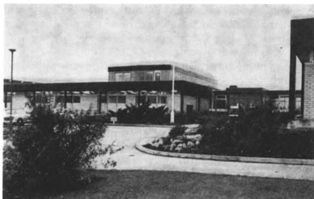
The Beecham Group's research centre at Harlow.
