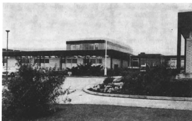
The Beecham Group's research centre at Harlow.
