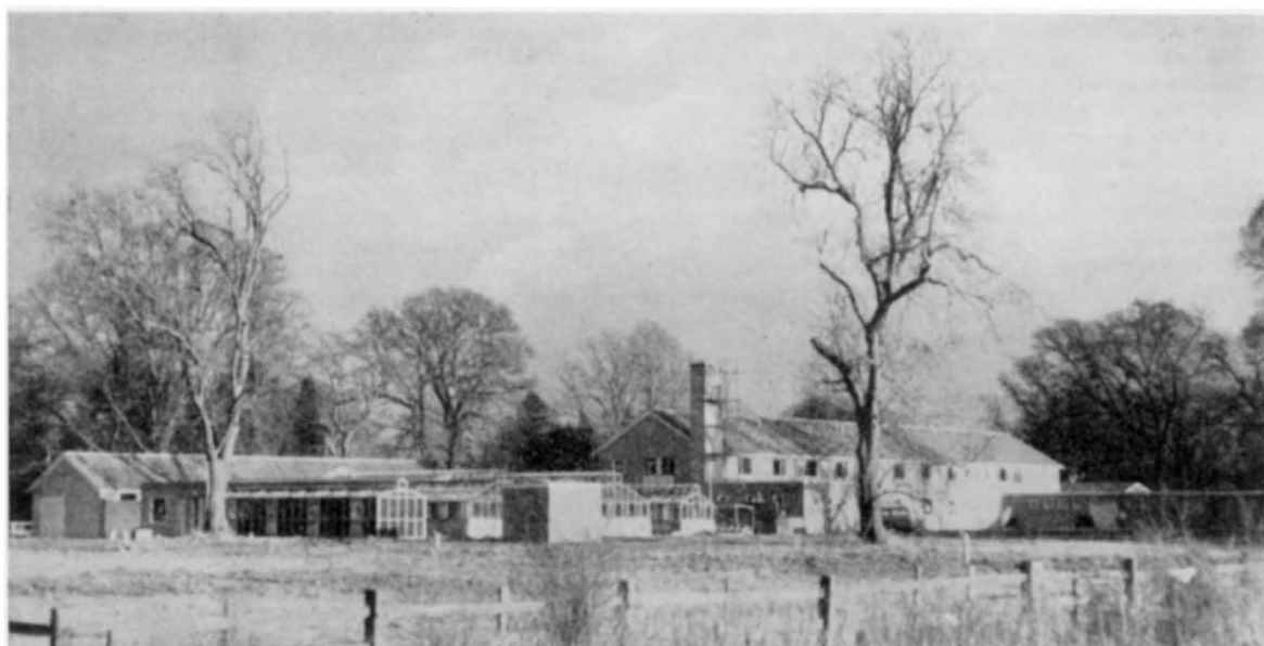
Fig. 1. General view of the Plant Pathology Laboratory, Harpenden, from the rear. (Photo by E. C. Large)
