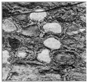
After saturation by rain, when drying takes place the lime forms into parallel lines with intermediate spaces, and those sand-grains which are thus robbed of their cement are speedily removed by the wind. The accompanying photograph (Fig. 1) is of an old stable wall built of local sandstones and limestones at the Military Arms Inn, The Nothe, Weymouth, and was taken in 1904. The scale is 1/10. I presume the cracks, etc., in old oil paintings are also quite unlike either of the above.
