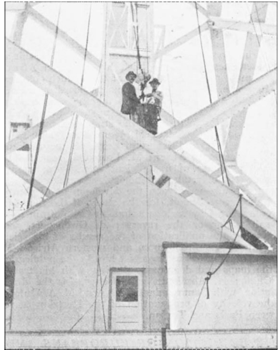
FIG. 2.—The observing house is directly below the tower and above the spectroscopes, which are situated in a deep vertical pit in the mountain.
