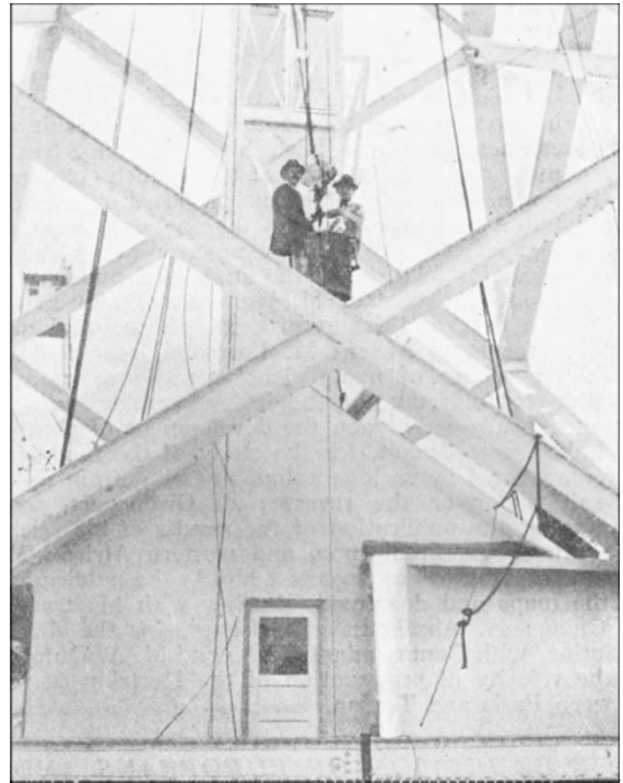
FIG. 2.—The observing house is directly below the tower and above the spectroscopes, which are situated in a deep vertical pit in the mountain.
