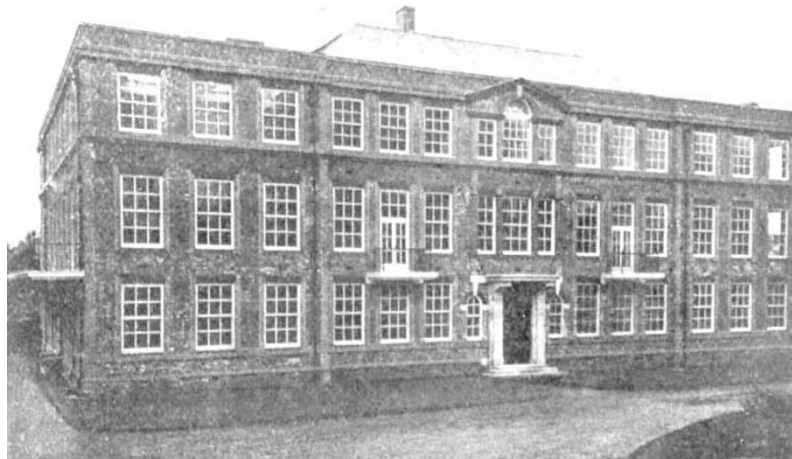
New building of the National Physical Laboratory.
