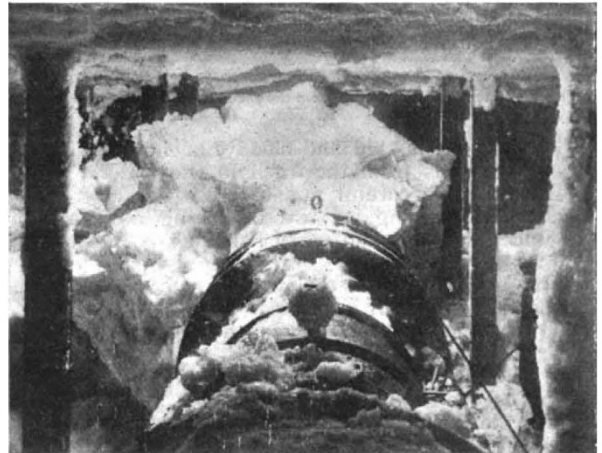
FIG. 1.—Interior of a penstock or wheel pit after the water has been removed, showing the accumulation of adhesive frazil ice.
