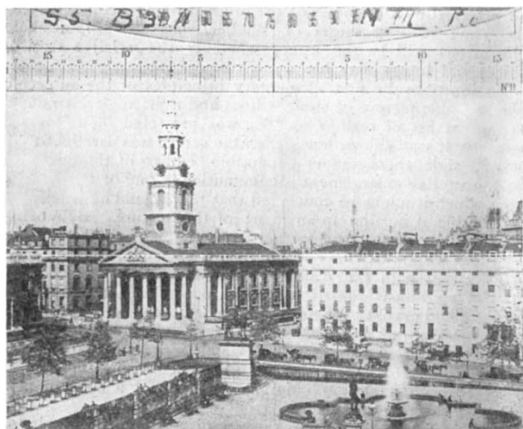
FIG. 2.—View from corner of roof of Union Club overlooking Trafalgar Square.
