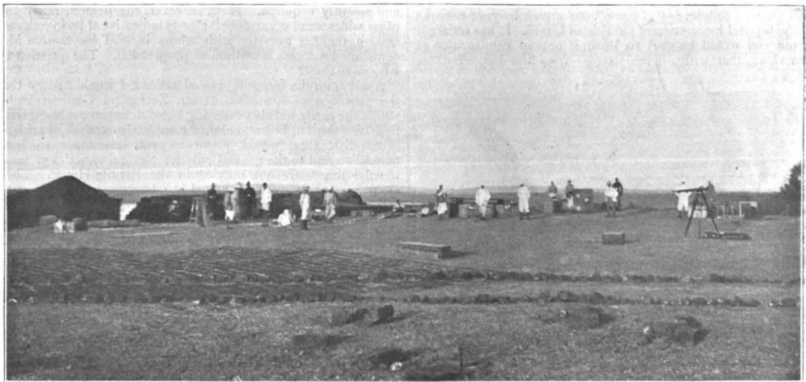
FIG. 1.—Camp, Saturday, January 8. Putting in concrete pillars.
