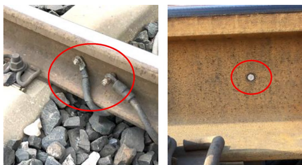
Figure 23. Grounding holes for simulating defects.
