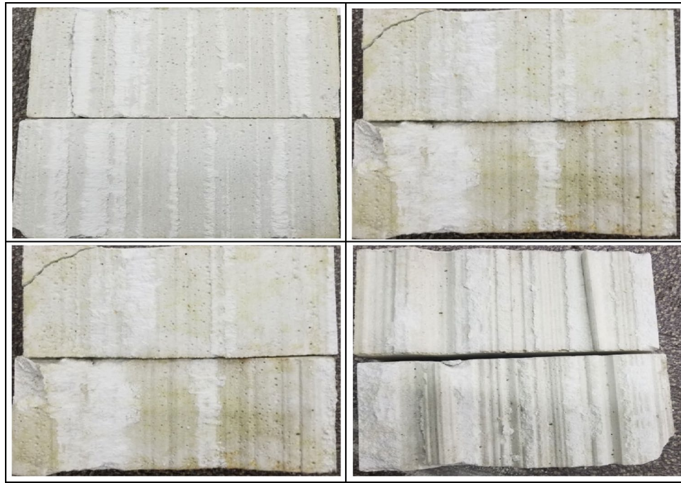
Figure 9. Surface damage of jointed rock mass.
